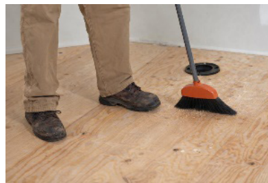
4. Prepare and clean subfloor
