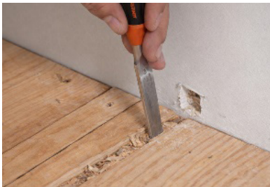
3. Install floor temperature sensor in conduit
