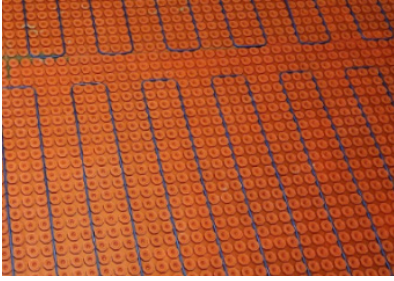
4. Lay heating cable (do not cut or cross)
