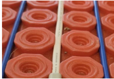
7. Lay the floor sensor cable into the mat equidistant from the cable
