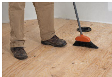
4. Prepare and clean subfloor
