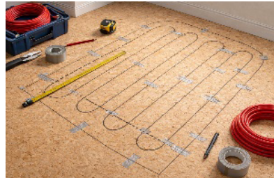
2. Mark the layout on the floor
