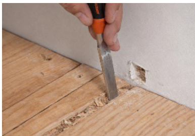
3. Install floor temperature sensor in conduit
