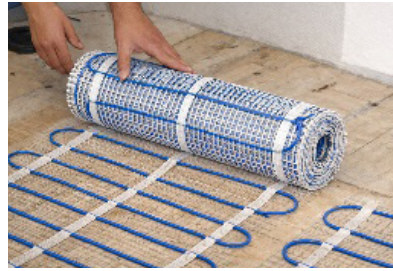
6. Lay heating mat
